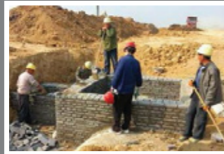
Collector Wells, Biochemical tank liquid level detection
